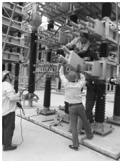
图9 电容器更换装置应用某市 \pm 800 kV 换流站检修 Fig. 9 Application of capacitor replacement device for maintenance of Shenzhen \pm 800 kV Dongfang converter station
